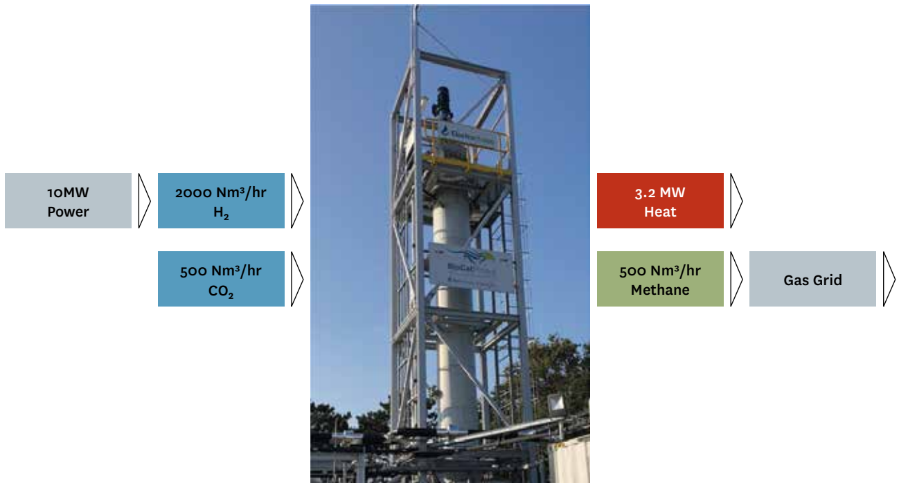
A 10 MW biomethanation plant could produce up to 500 Nm 3 /hr methane and 3.2 MW heat
