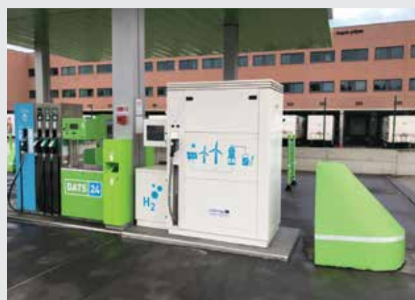
The Colruyt integrated refuelling facility demonstrates the hydrogen refuelling hub model of distributed generation powering facilities, producing hydrogen with the excess power and fuelling both forklifts and trucks and cars at different refuelling points.
