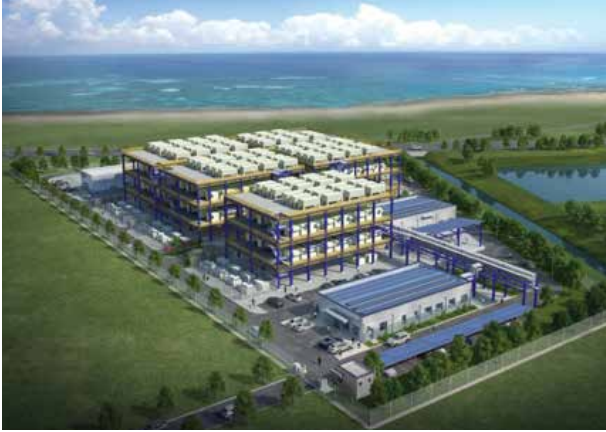
Hanwha Energy and Korea East-West Power have started construction on the world's first 50 MW hydrogen fuel cell power plant. The plant is expected to cover over 20,000 square meters and provide 40,000MWh of energy per year, enough to power 17,000 thousand households. Construction is scheduled to be finished by 2020.
